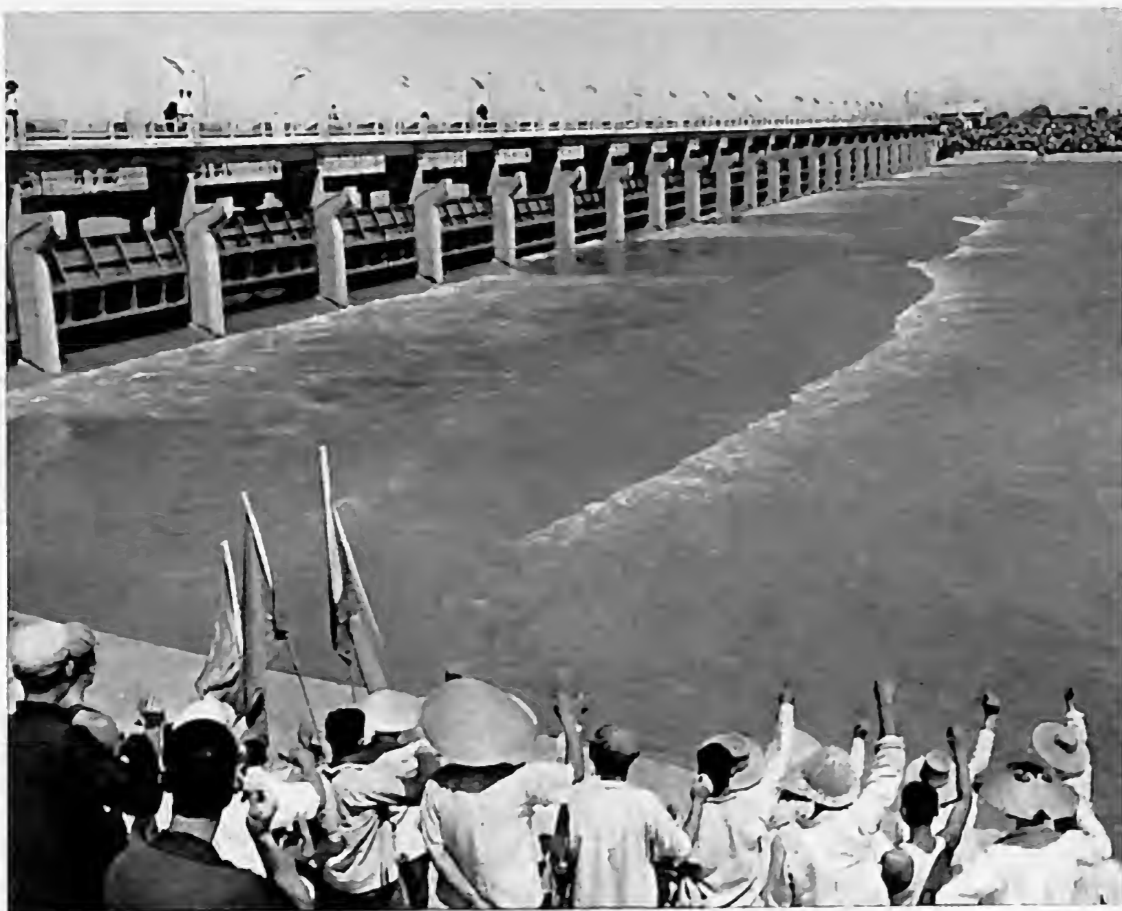
The Tsaolinchuang junction project on the Taching River near Tientsin. Harnessing the river has freed farmland on the banks from flood and waterlogging.
